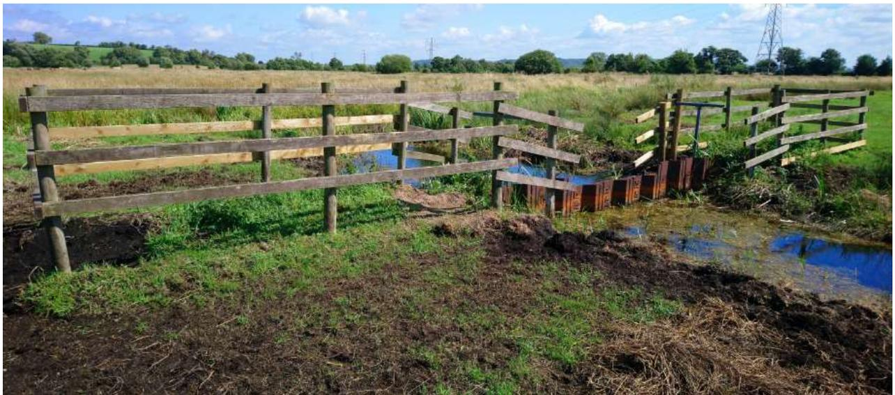
*Pictured above: completed Trench Sheet Dam at Moorlinch*
