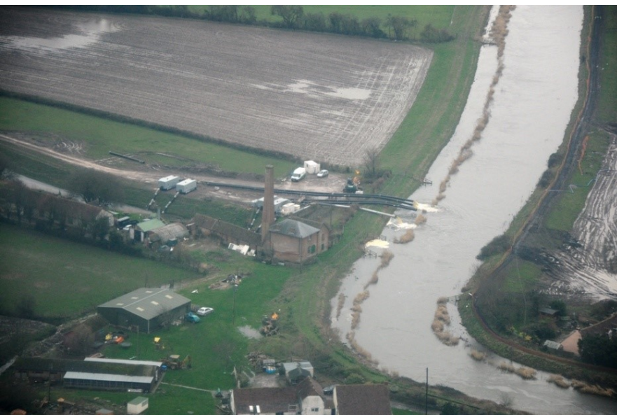
Westonzoyland pumping station and additional pumping
