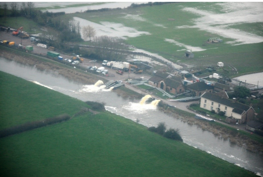
Northmoor pumping station and additional pumping
