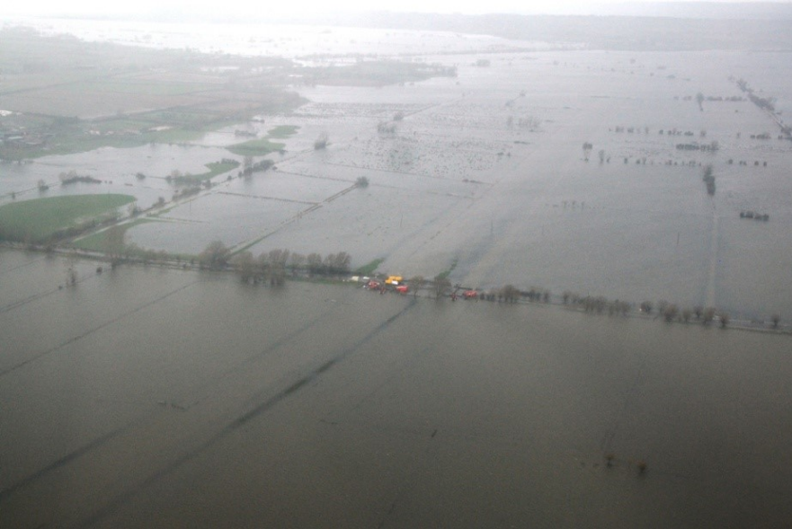
Photo shows A372 at Beer wall and additional pumping before improvements were made after 2013-14 flooding.
