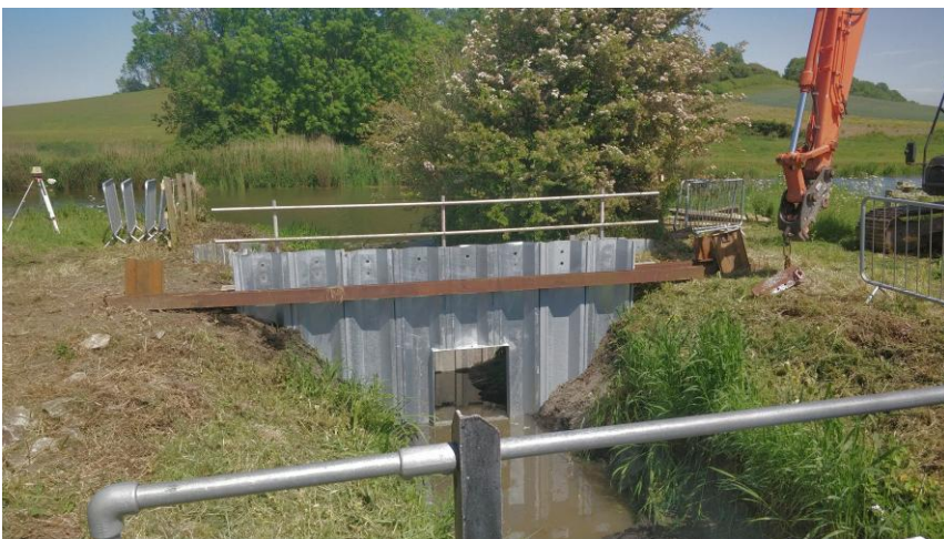
Chedzoy Tilting Weir: Flap Valve Sheet Pile Headwall
