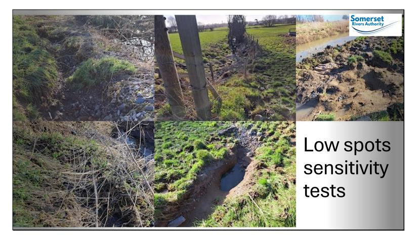
Aware of localised bank erosion resulting in preferential overtopping. Concern that filling in these low spots could make flooding worse somewhere else, so needed to be assessed in the model.
