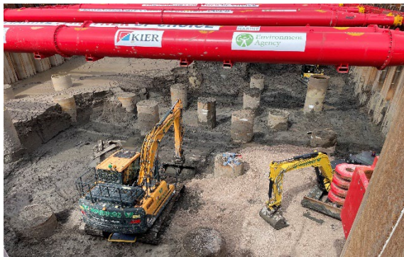
Plate 2-Working inside the central cofferdam with the tubular piles.
