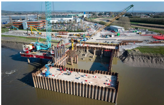
Plate 1-Construction of the Barrier substructure
