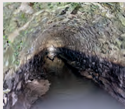
Inside a siphon
