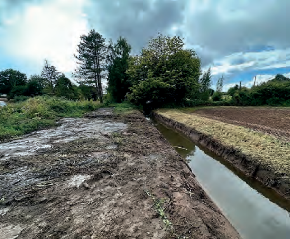
Left: Watercourse desilting works completed to help reduce flooding in Asham Lane, Ham
